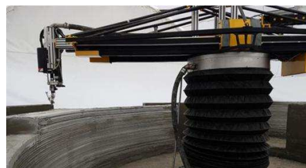
3D Printing - Construction
